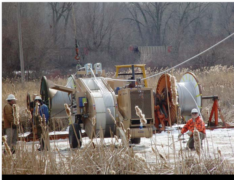
Setup with 3M-recommended 3-to-1 breakover wire slope from the first dolly to the tugger and tensioner.
