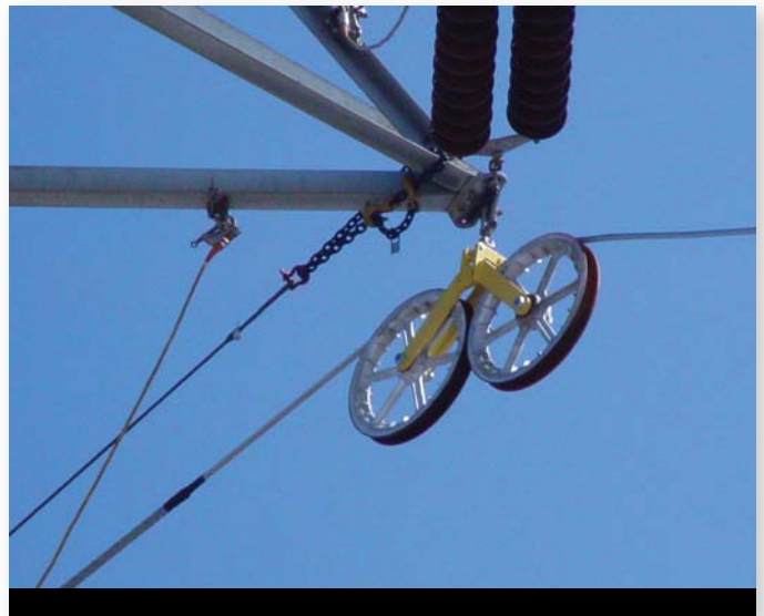
A double 28-inch sheave was used at the tensioning structure.
