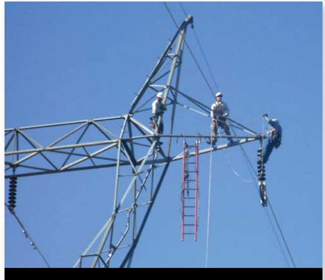
A line crews clips the conductor after stringing.
