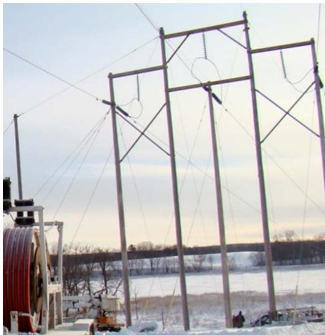
To get the results it needed within a tight 3 month time period, Xcel Energy chose to reconductor the line with 3M ACCR. As a result, it was able to keep the existing structures, cross a 1,570-foot (479 meter) span, and meet clearance and reliability requirements. Between November 2012 and February 2013, 3M developed and qualified a custom 183-T114 conductor for this application. The installation was done in just a few days.
