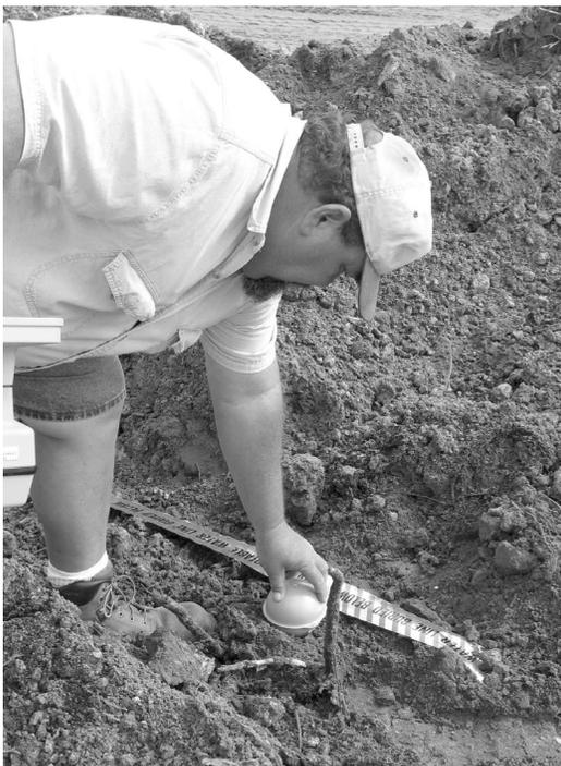
Witt places the 3M 1400 Series EMS iD Ball Marker in a water main trench to mark the pipe route before backfilling.
