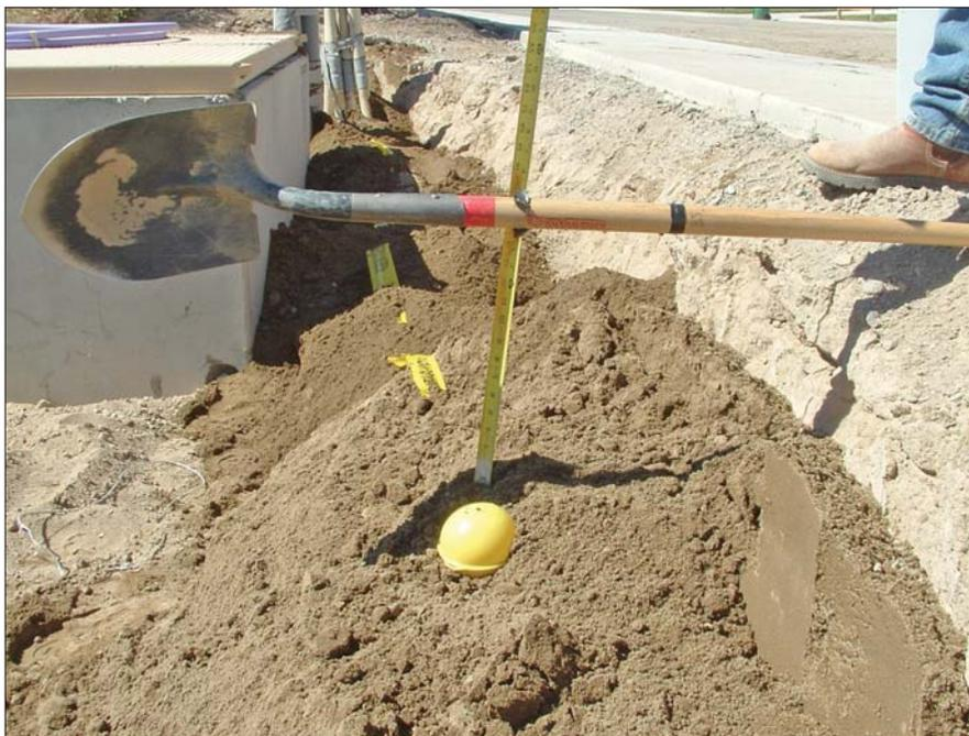
ments are sometimes difficult to find with traditional methods and we now mark them electronically as pipelines are installed or excavated for repair."
