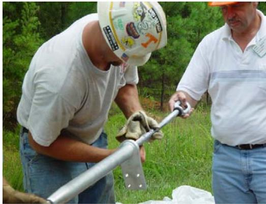
*Figure 3: ACCR larger outer sleeve, which is similar to conventional conductor accessories*
