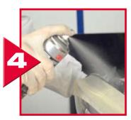
Coat tab area in 3M™ Polyolefin Adhesion Promoter 05917 and leave to dry for 10 minutes.
