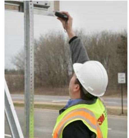
Above: scanning the sign barcode. Below: entering data into the sign management system.
